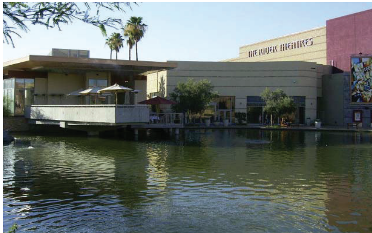
Figure 1 – C The multiple commercial uses planned for the Imperial Center are proposed to share a water feature and unified design
