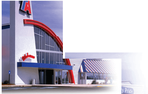
Figure 6 - C Convenience Store & Gas Station
