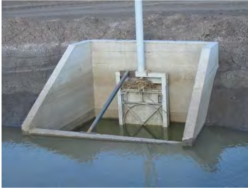
Photo 5-1: Weir Box precast delivery gate
